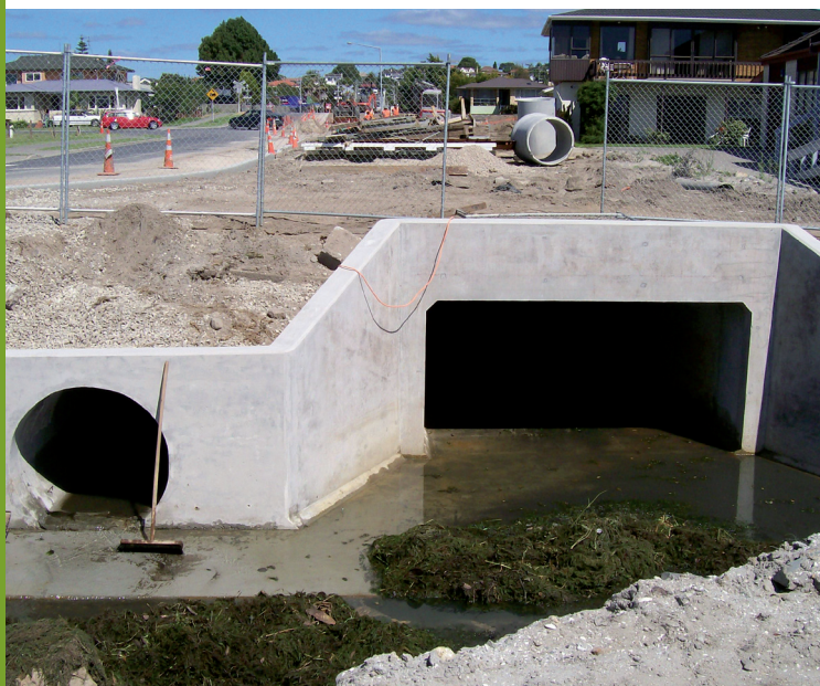
The stormwater upgrades on Bureta Road in March 2007. The open drain has now been piped and a culvert is in place.
